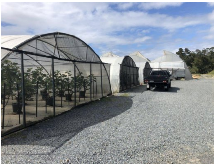
Photograph 3 – Looking south across greenhouses.
